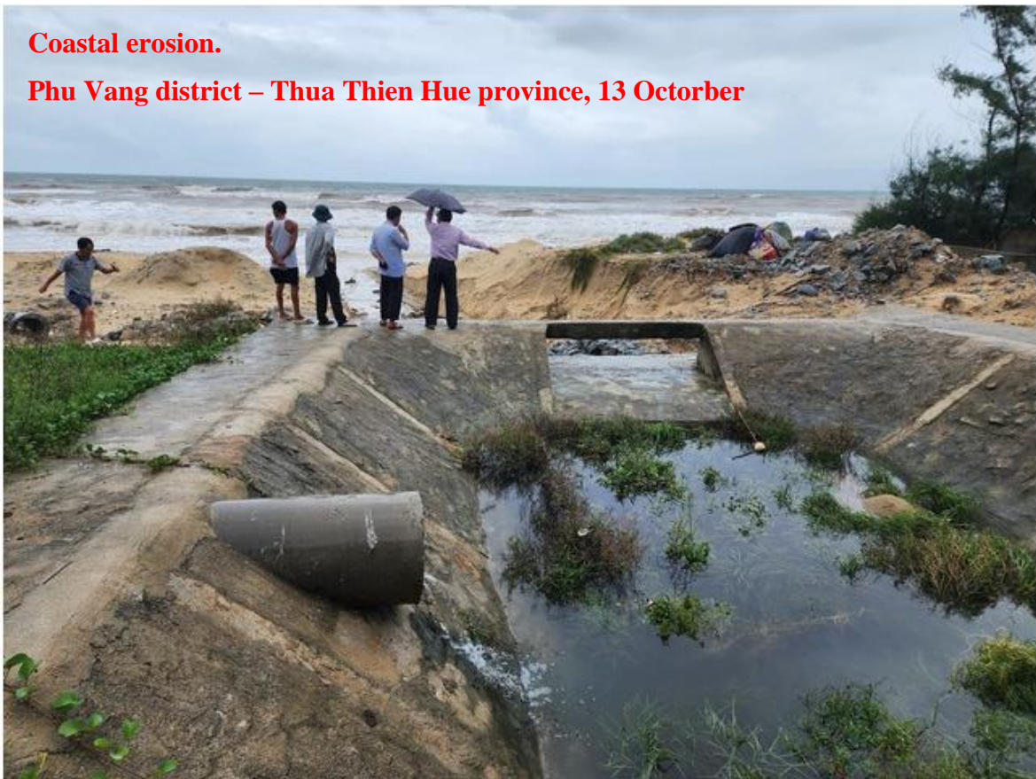
Figure 2.5. Flooding and coastal erosion in Thua Thien Hue provinces
